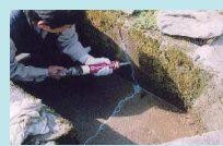
ひび割れ補修
